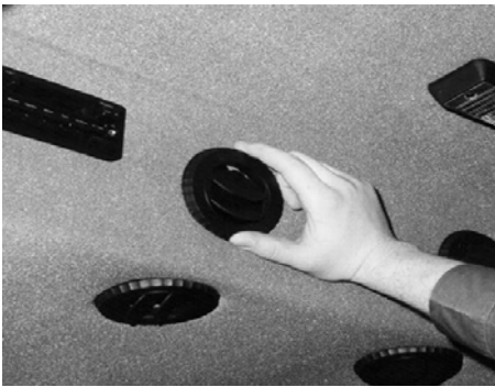
Air Vents -Typical View
