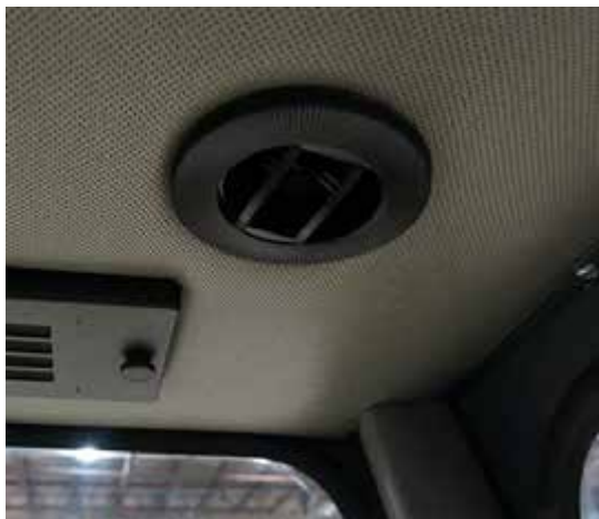
Air Vent -Typical View
