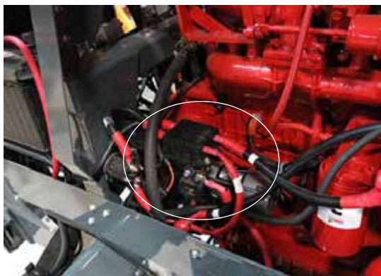
Wire Harness Circuit Breaker and Fuses (Located on the right-hand side of engine) -Typical View
