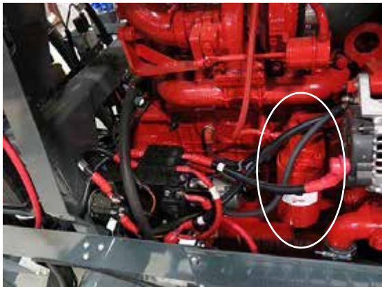
Engine Oil Filter (Located on the right-hand side of engine - open hood panel to access) -Typical View
