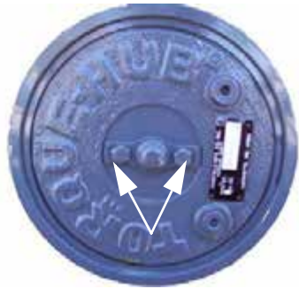
Cap Bolts -Typical View
