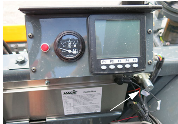
Traction Valve Switch - Front (Located near the front of operator's station) -Typical View
