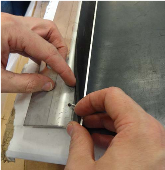
Brush Curtain Assembly -Typical View
