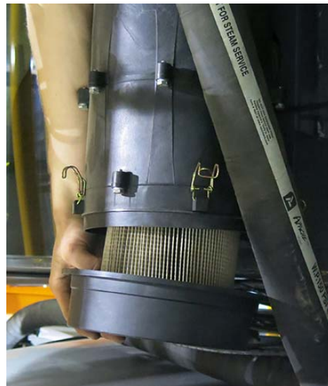
Filter Removal -Typical View
