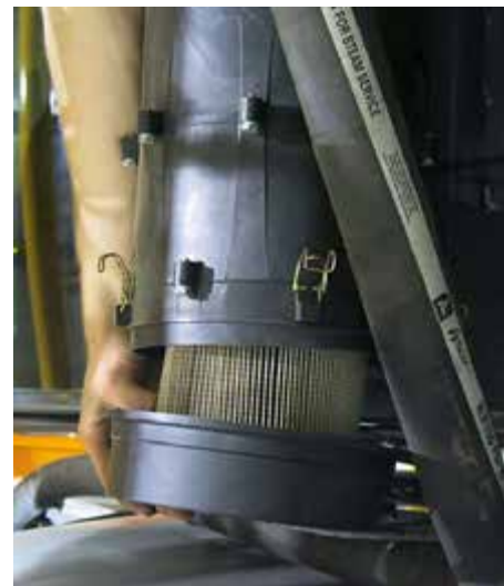
Filter Removal -Typical View
