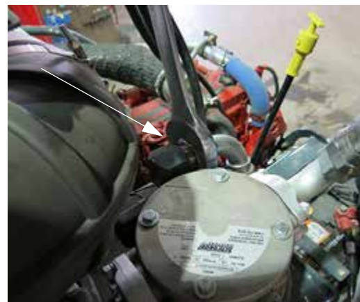
Case Drain Hose (Located near top of hydraulic reservoir) -Typical View
