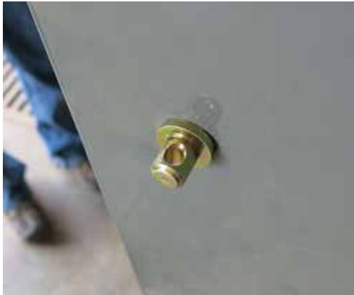
Hanger Pin Installation -Typical View
