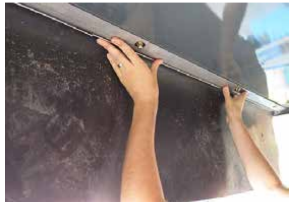
Brush Curtain Installation -Typical View
