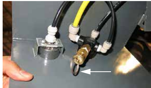
Pressure Relief Pull Ring (Located on the back side of the foam pressure regulator) -Typical View
