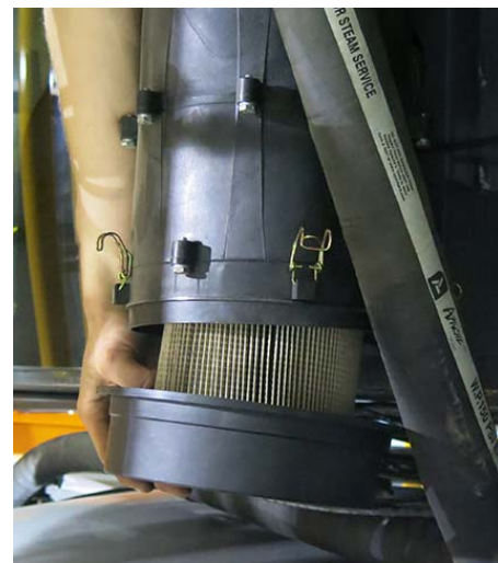
Filter Removal -Typical View
