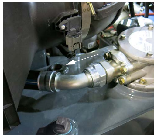
Breather Cap Removed -Typical View
