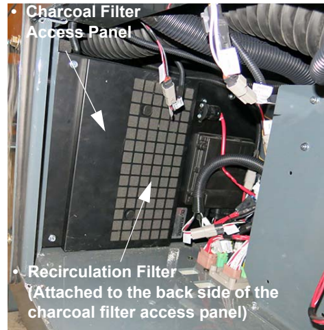
Charcoal Filter Access Panel (Located behind exterior service panel on right-hand side of cab) -Typical View
