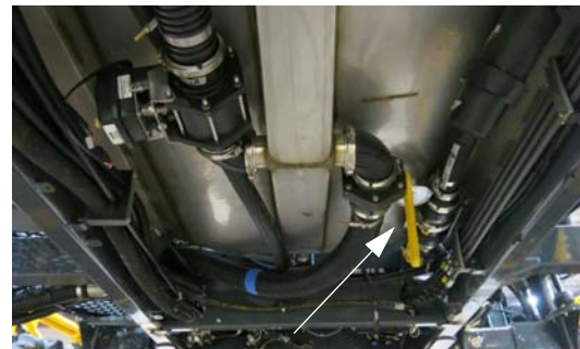
Sump Valve -Typical View
