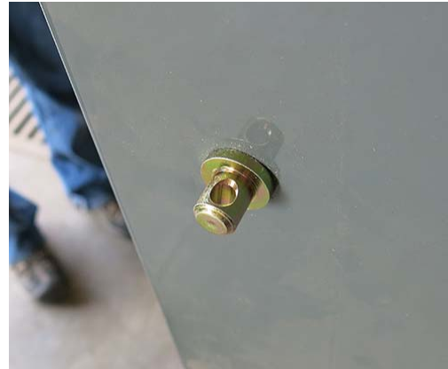
Hanger Pin Installation -Typical View
