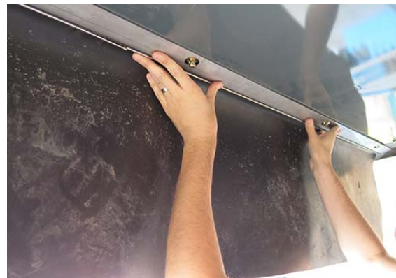
Brush Curtain Installation -Typical View
