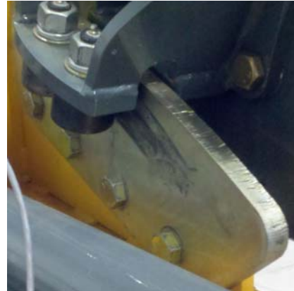
Friction Plate (Located in the bottom corners between the fixed transom and pivot transom) -Typical View
