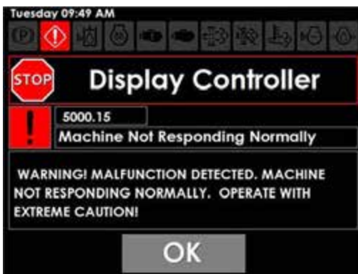
Machine Fault Warning
