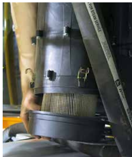
Filter Removal -Typical View
