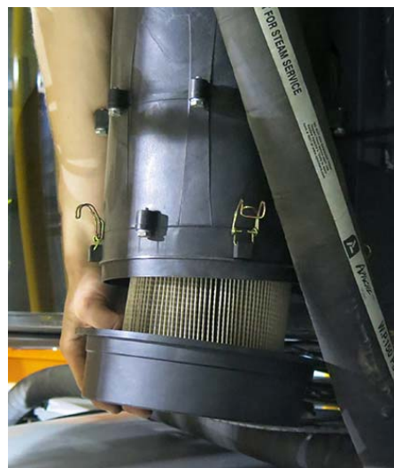
Filter Removal -Typical View
