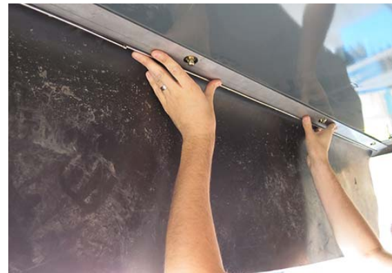
Brush Curtain Installation -Typical View
