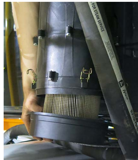
Filter Removal -Typical View
