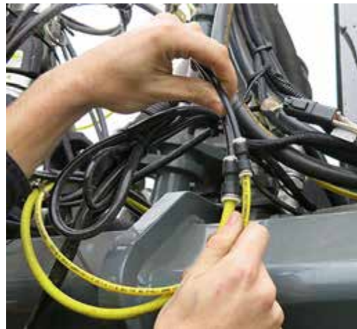
Foam Marker Connection (Located on the front right-hand side of machine) -Typical View
