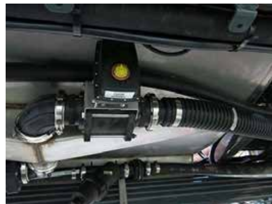
Solution Tank Valve -Typical View
