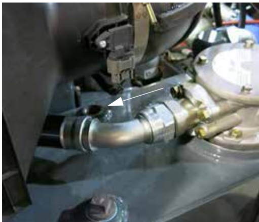
Breather Cap Removed -Typical View
