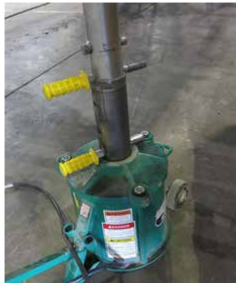
Lock Pin Installation -Typical View
