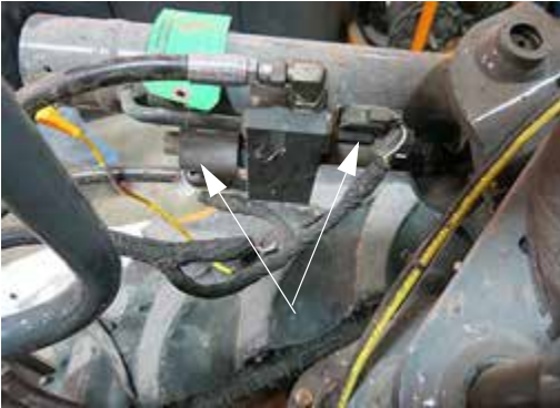
Lock Valves -Typical View
