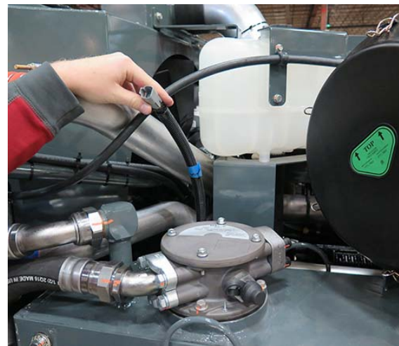
Level/Temp Sensor (Located on top of hydraulic oil reservoir) -Typical View
