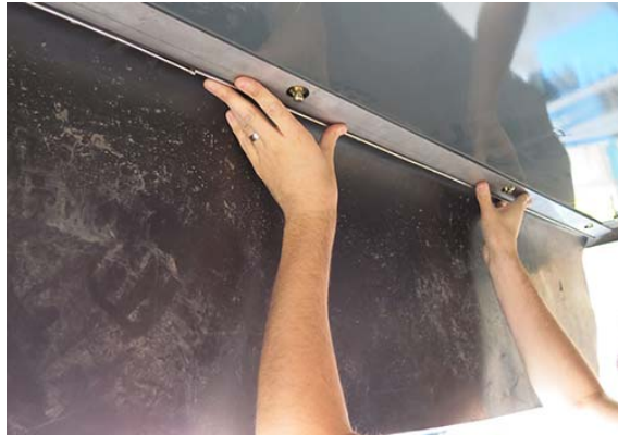
Brush Curtain Installation -Typical View
