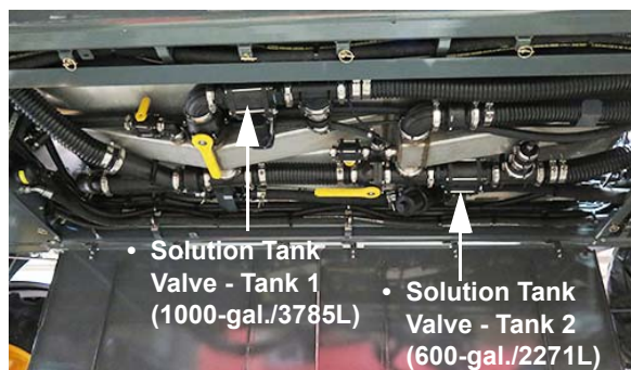
Solution Tank Valves - Tanks 1 and 2 (Located beneath the solution tank on underside of machine) -Typical View
