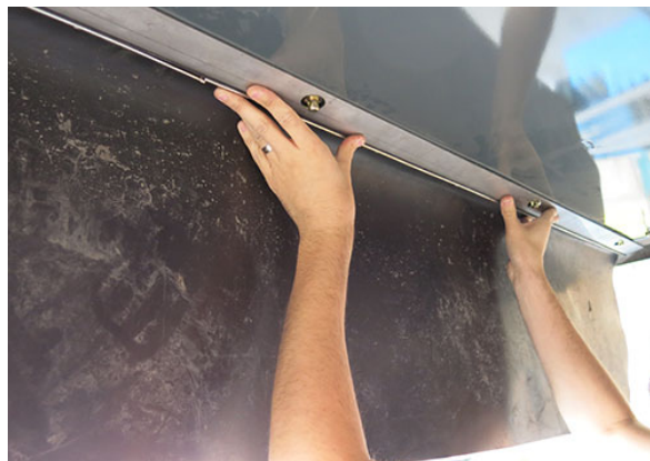
Brush Curtain Installation -Typical View
