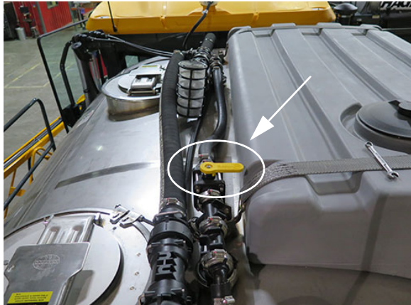
Dual Product Rinse Valve (Located on top of the solution tank) -Typical View
