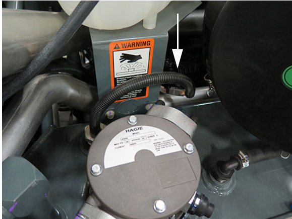
Level/Temp Sensor (Located on top of hydraulic oil reservoir) -Typical View
