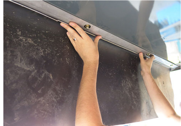
Brush Curtain Installation -Typical View
