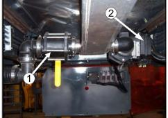
tank sump valve (fig. 4.52-2, item 2) is a ball type valve that has to be turned on and off manually.
