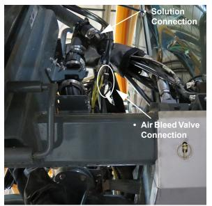
Solution and Air Bleed Valve Connections - **Standard**
