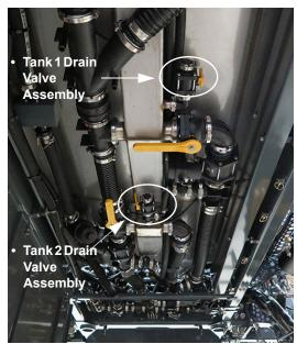
Solution Tank Drain Valve Assemblies (2)
